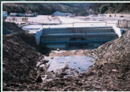
▲ The debris screen at the top end of Crumplehorn Car Park
