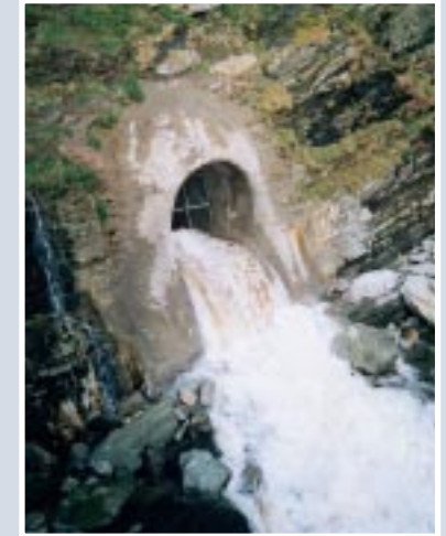
▲ The scheme in action: Floodwater discharging direct to the sea and out of harms way
